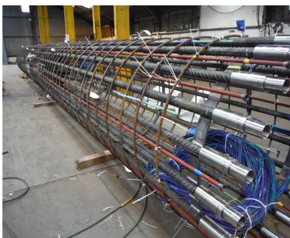
Figure 5. Assembly of the O-cell reinforcement cage inside the steel manufacturer's workshop.
