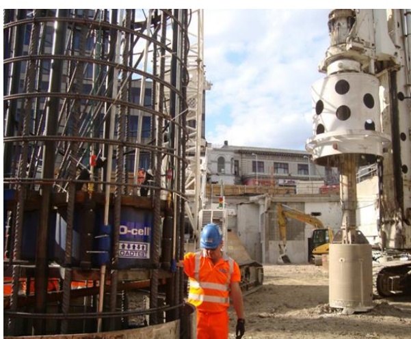
Figure 3. Cage and O-cell assembly installation at Farringdon station.
