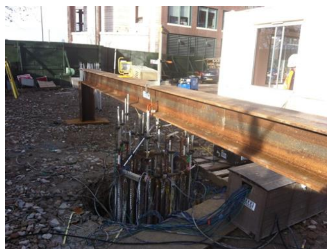
Figure 4. Reference beam over the O-cell test in progress at Canary Wharf.
